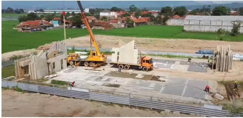
Figure 2. Precast House Panel Production
